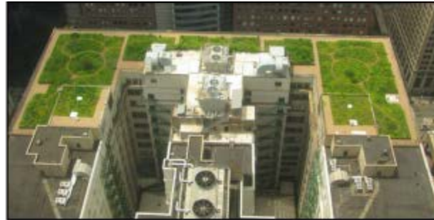
Green roof of City Hall in Chicago, IL.
